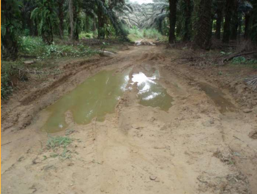
Unsafe and bad road upkeep
