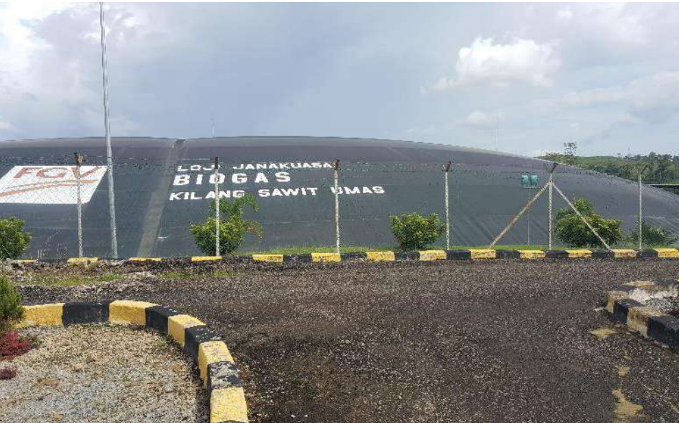
Engineered lagoon AD
