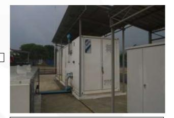
1<sup>st</sup> stage compressor unit and membrane separation system
