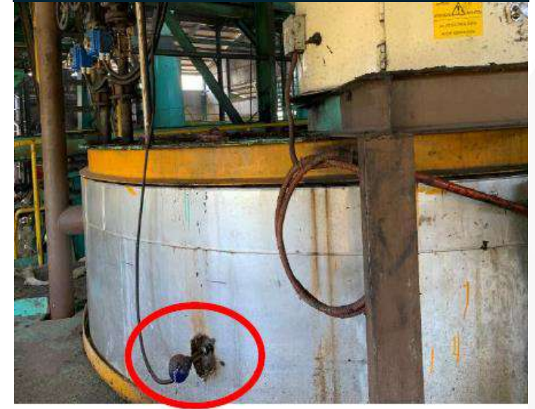
Temperature Transmitter
