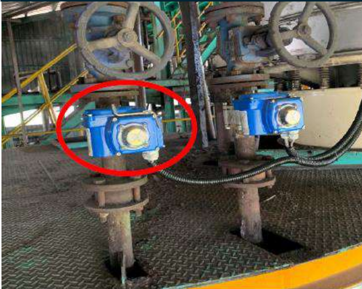
Steam Inlet Control Valve - VCT
