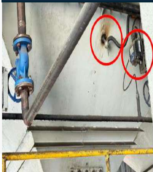
Steam Valve and Temperature Transmitter
