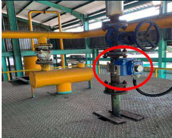
Steam Inlet Control Valve - VCT
