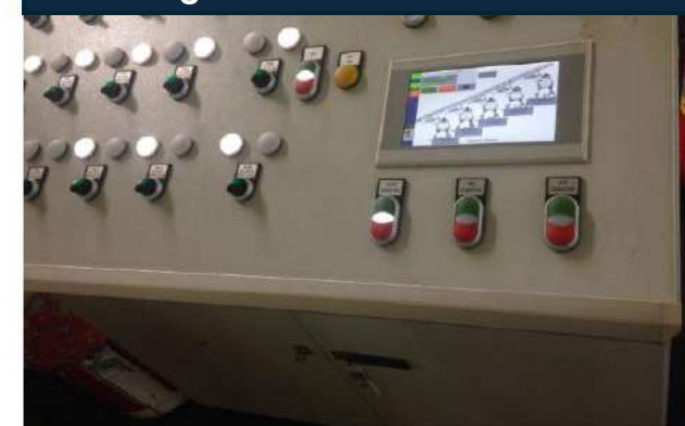
Digester Level Control Panel
