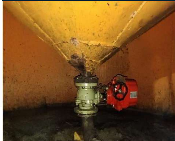
Drain Control Valve
