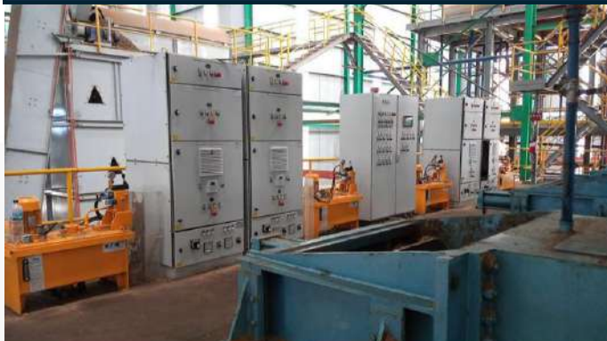
3 in 1 Panel (Screw Press with Inverter)
