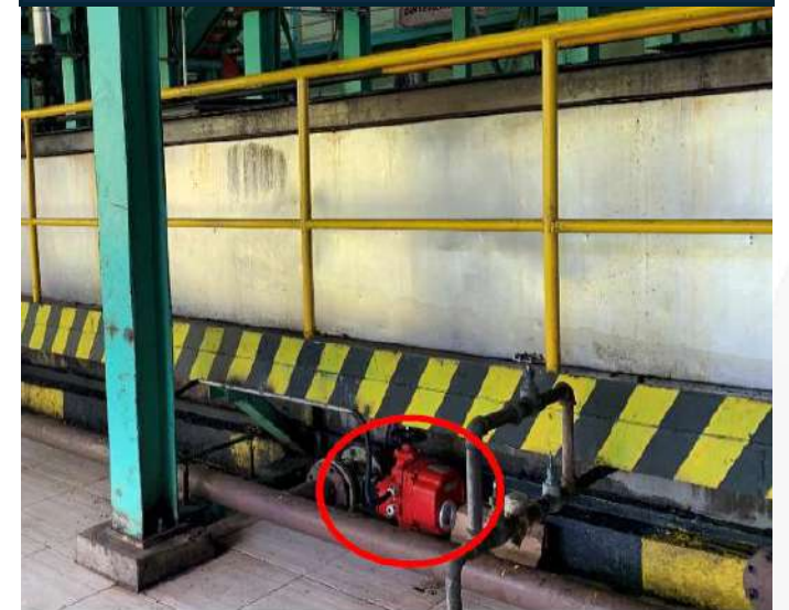
Drain Control Valve
